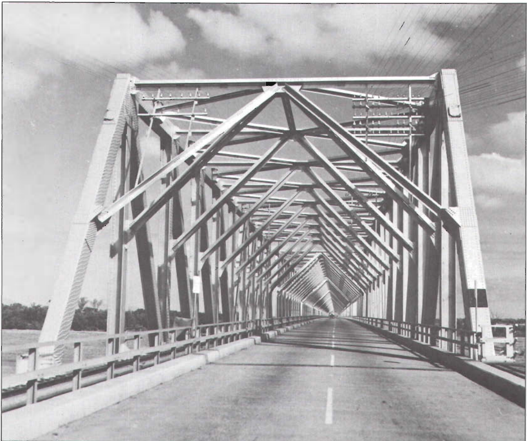
Burdekin River Bridge
